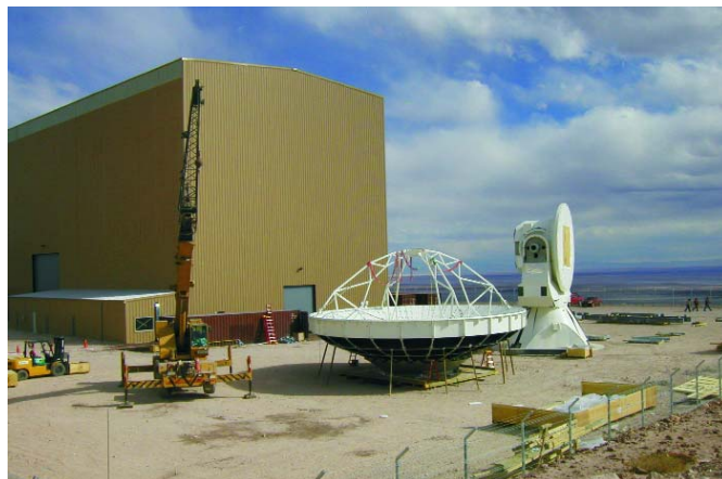
Figure 2. The first ALMA production antenna at the OSF: the VertexRSI pedestal stands on its pad to the right of the partially assembled backup structure, and in front of the VertexRSI site erection facility.
